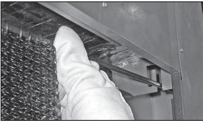
Figure 15.12 Place Right End of Screen Rod
